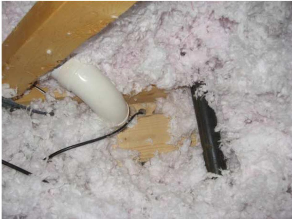
I drilled a hole through a joist (I hope it wasn't supporting anything too important) and ran the coax cable through it. I elected to use RG-58 for its availability, easy installation and sufficient performance for this application. In this picture, the black RG-58 can be seen running on the right side of the white PVC pipe.
